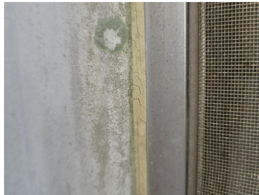
3104-12 Caulk (5% Chrysotile) Typical Exterior Doors/Windows
