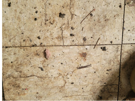
3104-8 12"x12" Floor Tile (3% Chrysotile) Interior Utility Shed (Appx 30 sq ft)
