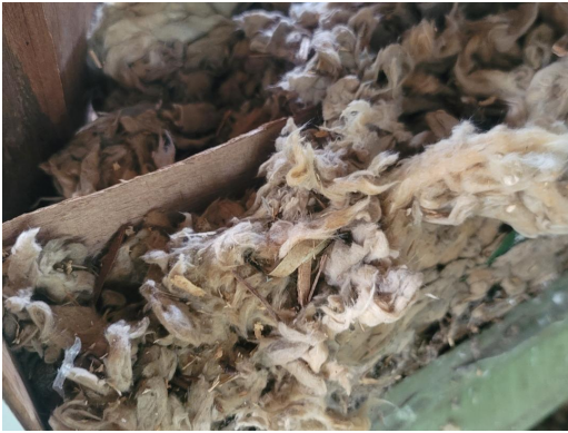
3104-1 Insulation Typical Interior
