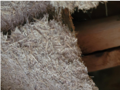
3104-3 Ceiling Material Typical Interior
