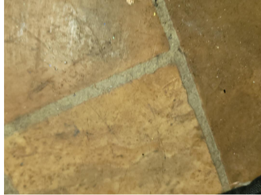
3104-14 12"x12" Floor Tile/Adhesive Interior Enclosed Porch (East)
