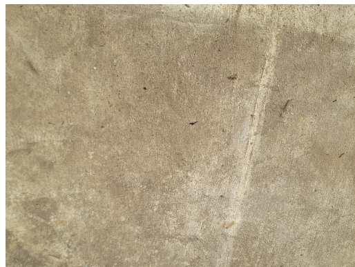
3104-6 Concrete Exterior Driveway/Sidewalk/Slab
