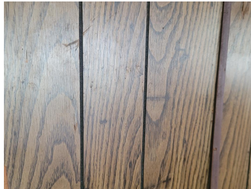
3104-4 Paneling Laminate Typical Interior Walls
