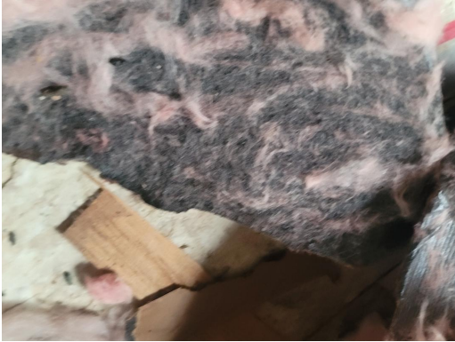
3104-7 Insulation/Mastic/Paper Interior Utility Shed
